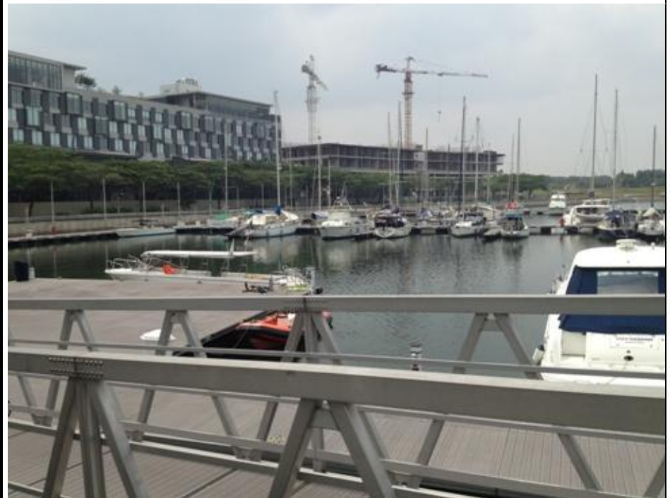
Figure 6: View from Puteri Harbour clubhouse: Traders Hotel completed while Somerset Apartments under construction
