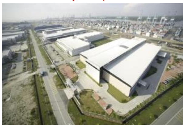
Figure 39: View of PFZ adjacent to port area
