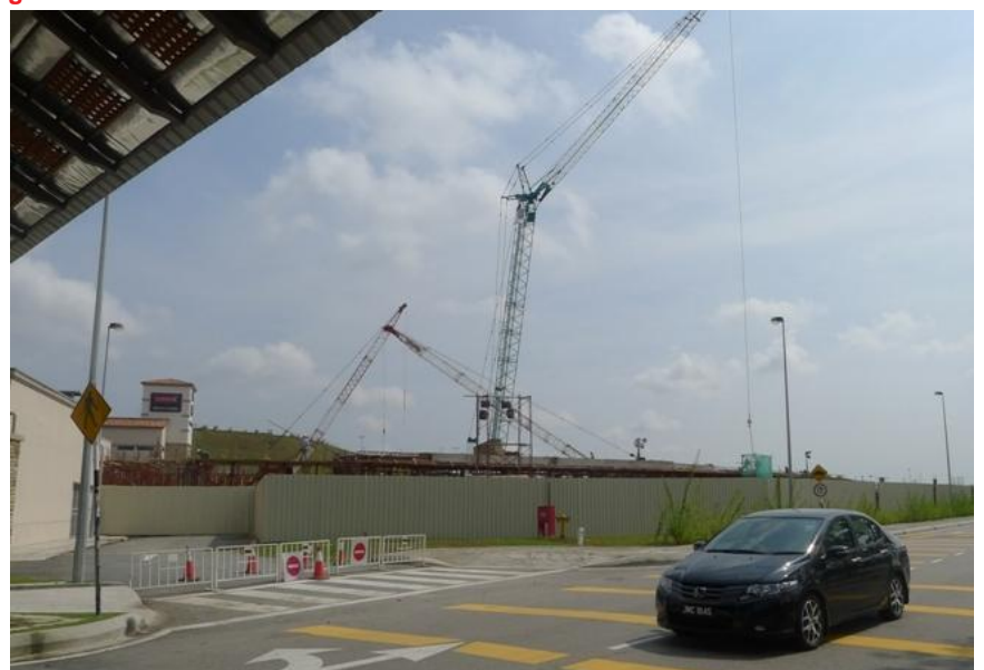
Figure 59: Construction works in JPO
